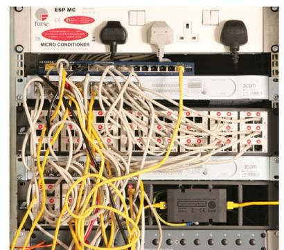
A Furse ESP Cat-5e/Gigabit (above and detail below) protecting a hub from transient overvoltages on a network connection with another building.
