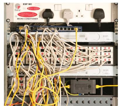
A Furse ESP Cat-5e/Gigabit (above and detail below) protecting a hub from transient overvoltages on a network connection with another building.
